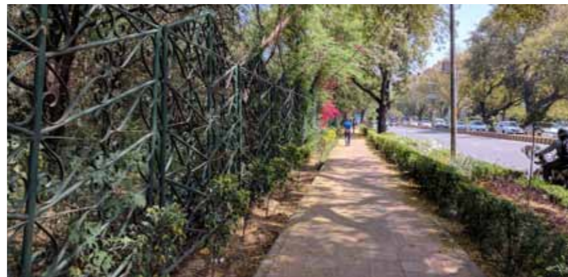
Boundary wall at Sardar Patel Marg
