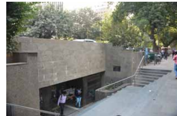
Wide entry to the subway allows for end to end view
