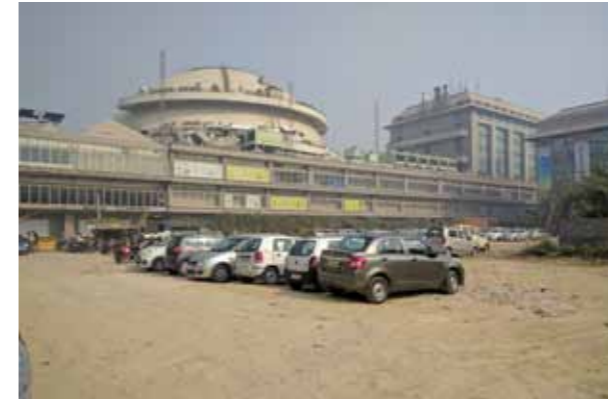
Unpaved and undulated space adding to dust
