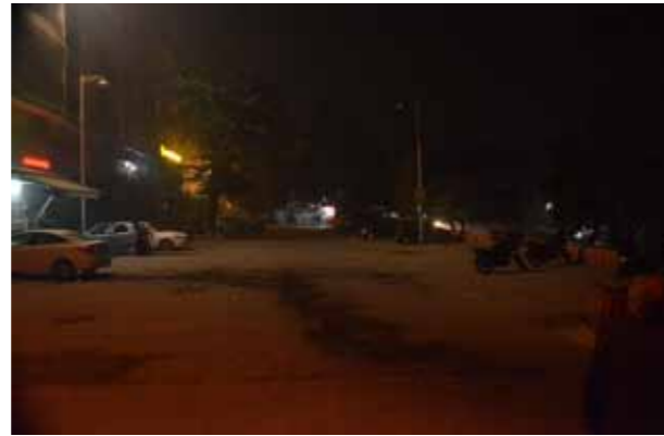
Defunct Light masts in Parking Lot
