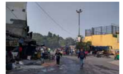
Absence of footpath along Urdu Academy
