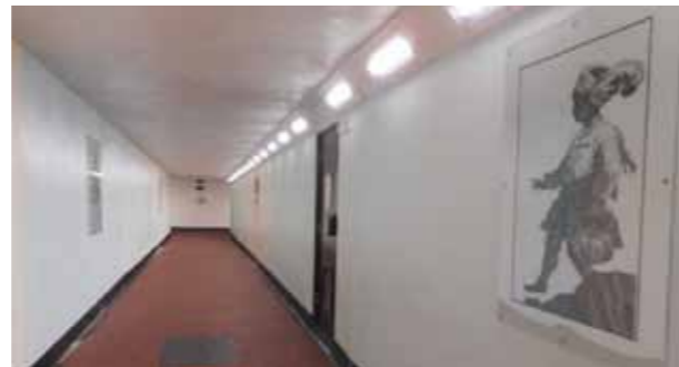
Proper lighting and artwork after renovation
