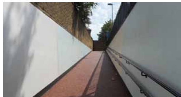
Entry after renovation
