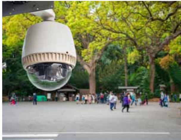
CCTV operating in outdoor park in Japan.
