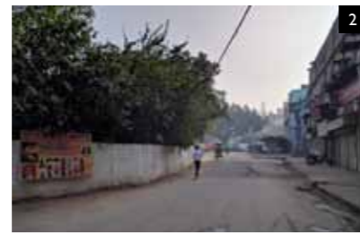
Absence of pedestrian walkway Urdu Academy, Church Road.
