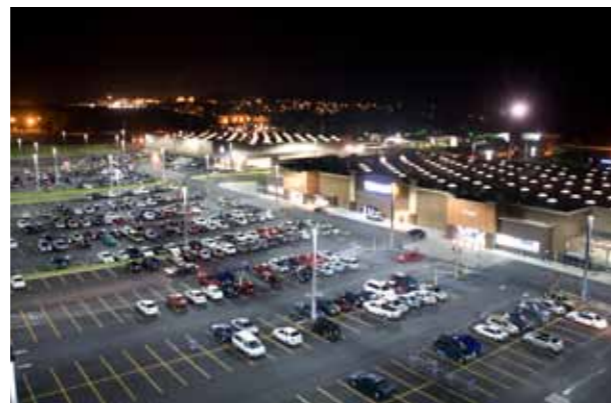
Lighting in Parking Lot
