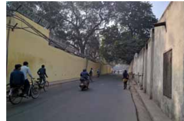
High boundary walls discouraging eyes on street
