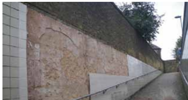
Entry before renovation
