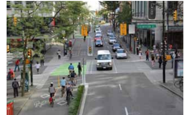
A complete street with a two-way protected cycletrack in Vancouver:
